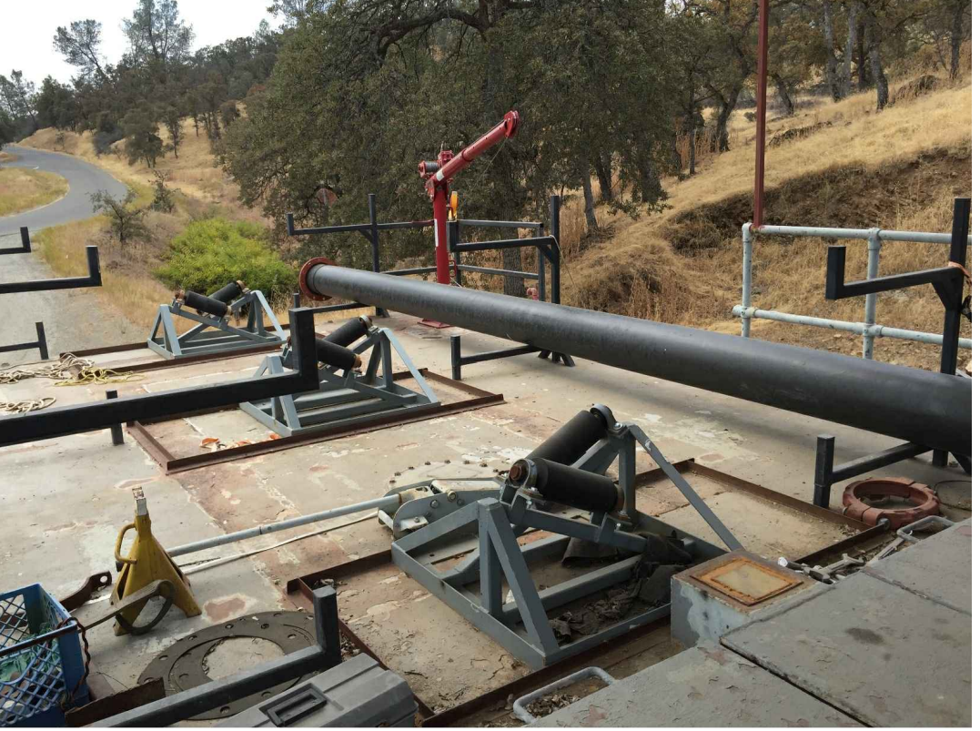
EXISTING BARGE PHOTO #4
